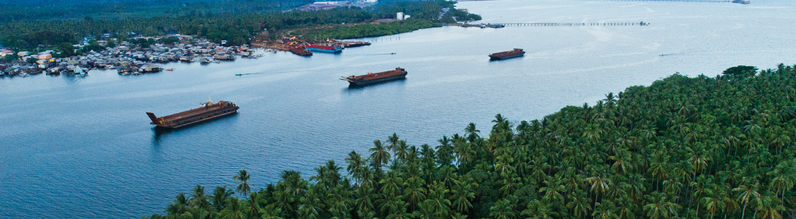
RTN - Loading Facility at the mouth of the Rio Tuba River
